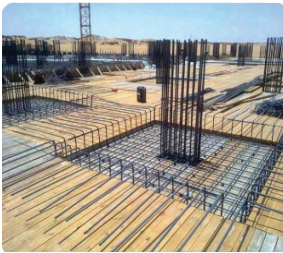
3 Shuttering and Reinforcement
