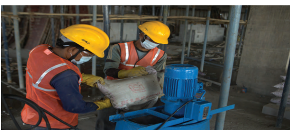
9 Grouting ( In Case of Bonded System )
