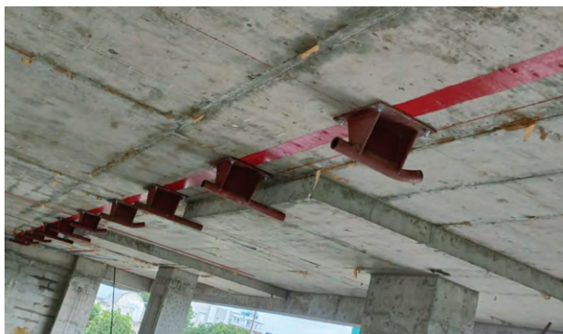
REACTION FRAME INSTALLATION
