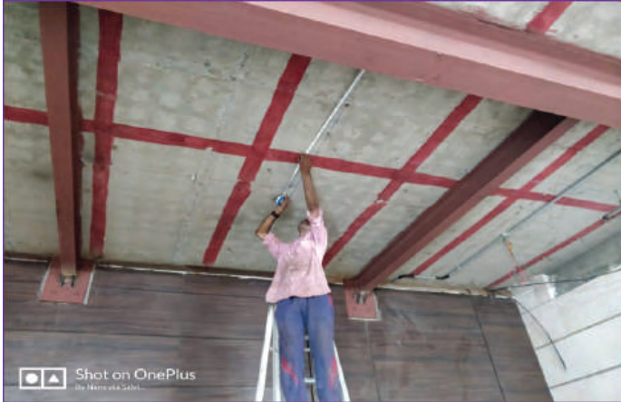
1. SLAB STRENGTHENING
