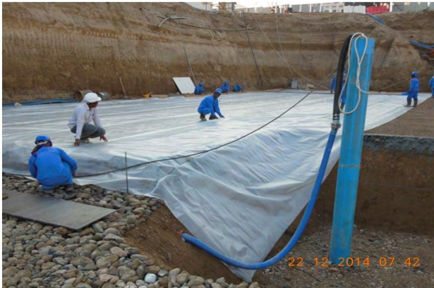
3. PLASTIC SHEET PLACING
