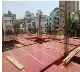
3 Shuttering and Reinforcement
