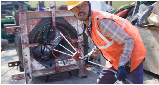
1 Decoiling of Cable
